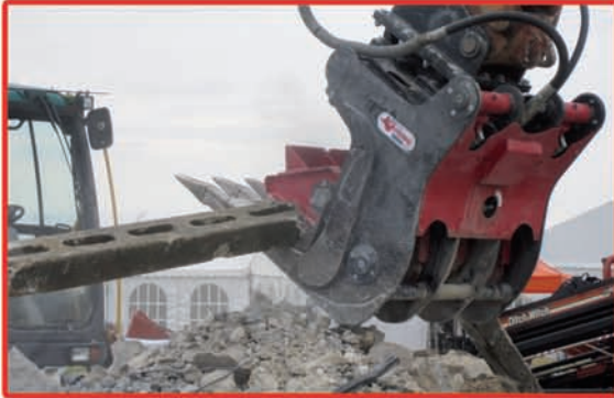
Breaking long precast beams with reinforced steel
